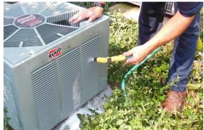
garden hose, spray water on and through the unit, washing the dirt and grime off the fan and coils, cleaning the fins, and removing any debris – like leaves or cut grass – that may have become lodged in the unit. If desired, you could also use a foaming coil cleaner (sold at most hardware
