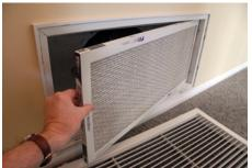
not run the air conditioner while you have the air filter removed. If you have the kind that can be washed and reinserted – such as an electrostatic air cleaner – make sure it is completely dry before re-installing it. If you have spring and summer allergies, buy the air filters with the highest MERV rating you can find, as they will filter out more pollens, mold and dust particles, and give you higher quality indoor air.
